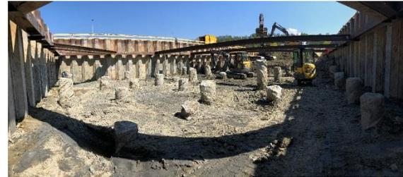
An existing silo stands 5 to 10 meters behind the excavation. According to the engineers, the settlement of this silo has to remain smaller than 3.5 cm. A first deterministic computation with ZSOIL® yields a 4.0 cm settlement.
